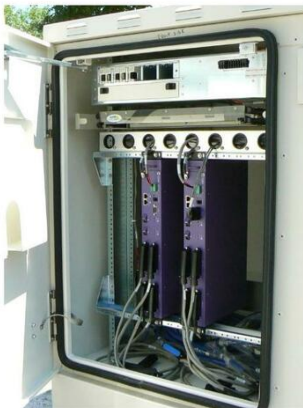
Calix ODC-1000ER; Remote Powered ODC-1000 Outdoor Cabinet with E5-110s
