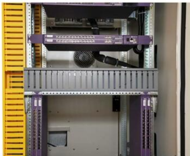
ODC-2000E/3000E Fiber Management detail (front view)
