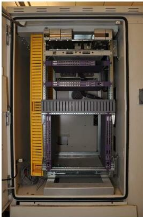
Calix ODC-2000E Outdoor Cabinet with E7-2s and Fiber Management Accessories
