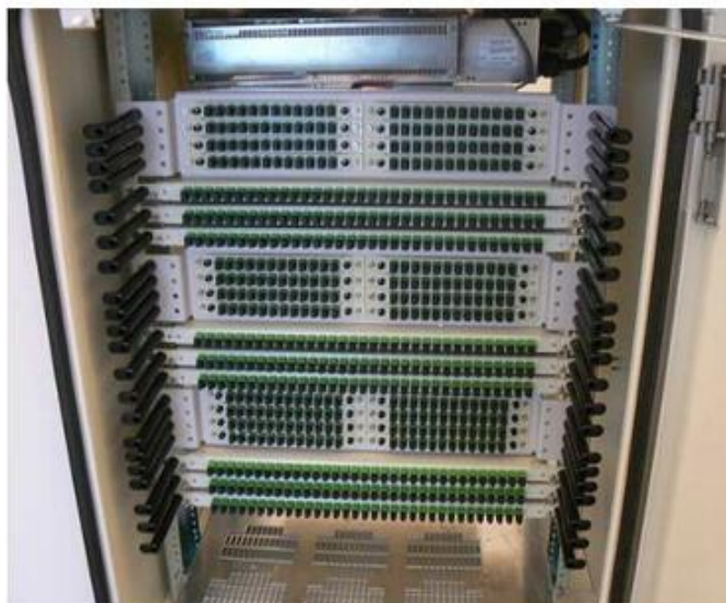
ODC-2000E with Fiber Management & Splitters
