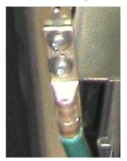
Figure C-10: Seismic Rack Ground Connection
