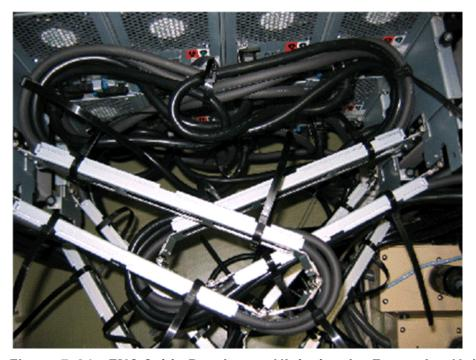
Figure 5-36: ENC Cable Routing on High-density Expansion Unit
