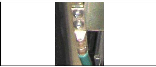
Figure 6-3: Seismic Rack Ground Connection
