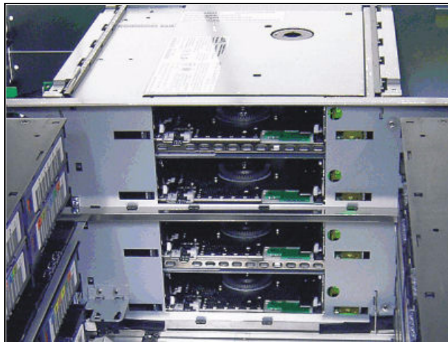
Figure 9-6 Interior of the TS3200 with four Ultrium 3 Half-High drives installed
