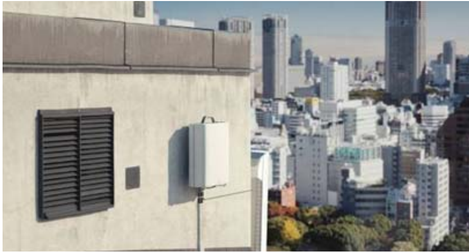
Figure 3-40: RBS 6302 typical installation
