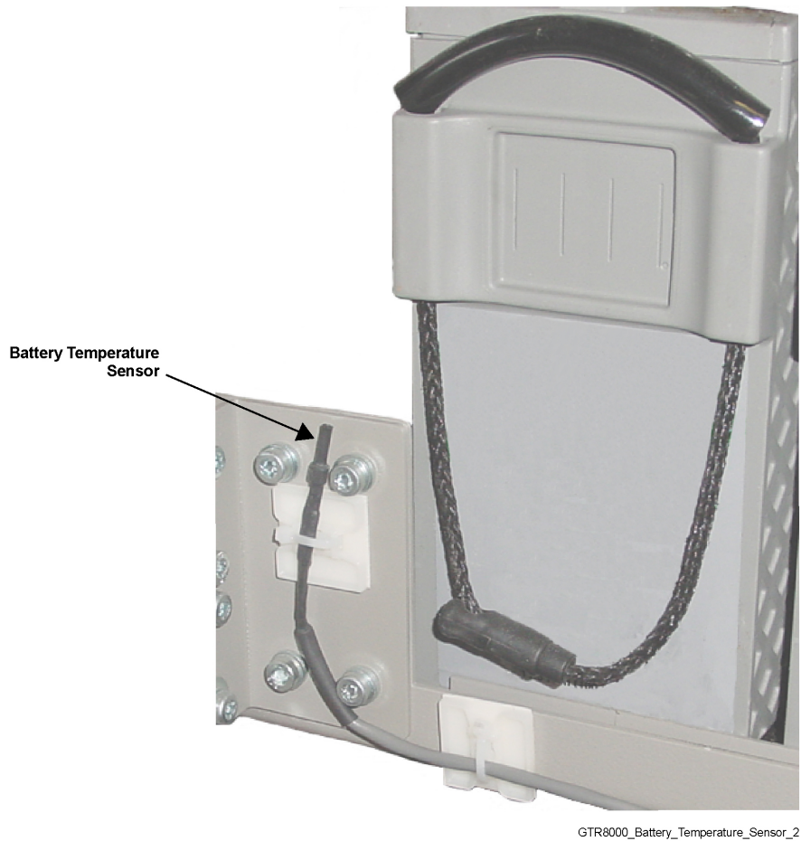
Figure 34: Battery Temperature Sensor Example 2
