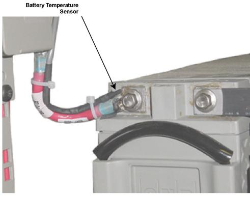
Figure 3-6 Battery Temperature Sensor Example 1
