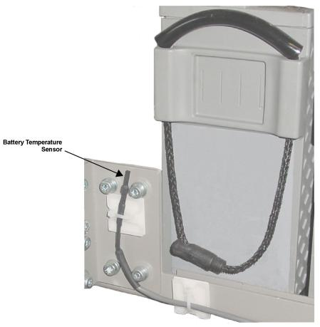
Figure 3-7 Battery Temperature Sensor Example 2
