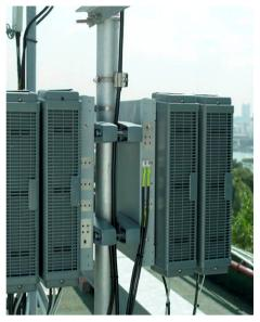
Figure 45: Installation options: Pole installation of Modules
