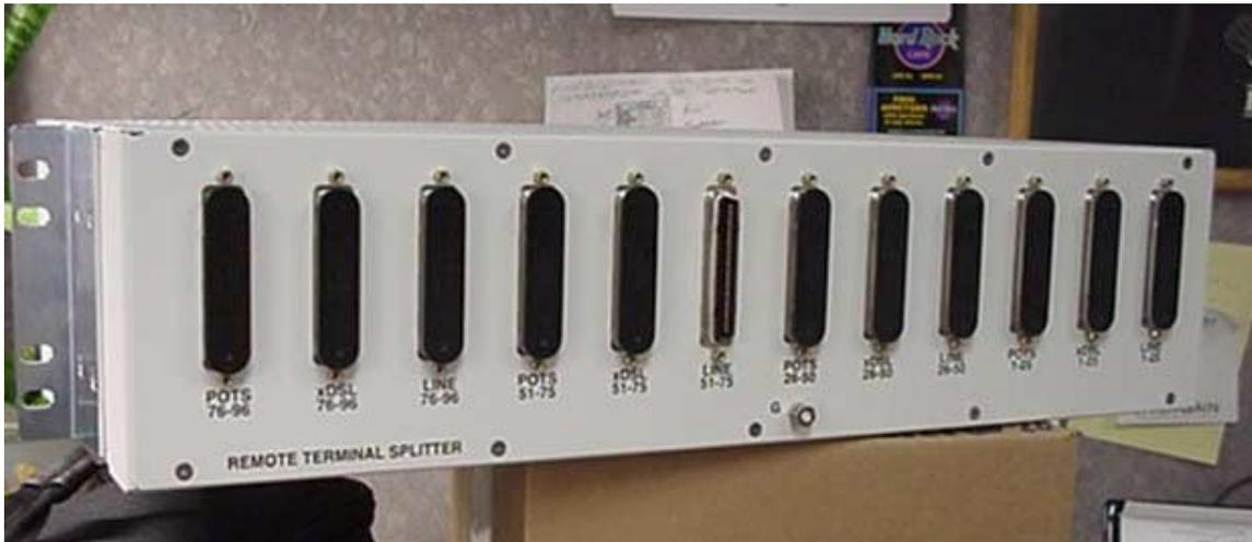
Notice the picture amphenol arrangement above. The AMP connections alternate Line, xDSL, POTS for OE, DATA, CP terminations. The count is sequential 1-96 on the frame blocks.
