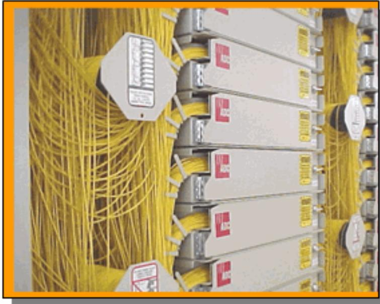
Illustration of the Generation III panels in the closed configuration
