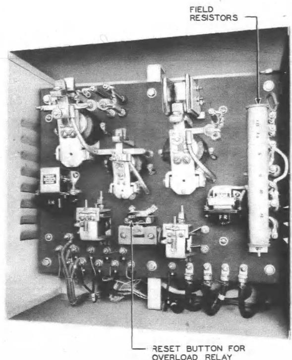
Fig. 1 - KS-5647, List 4 Motor Controller Front View
