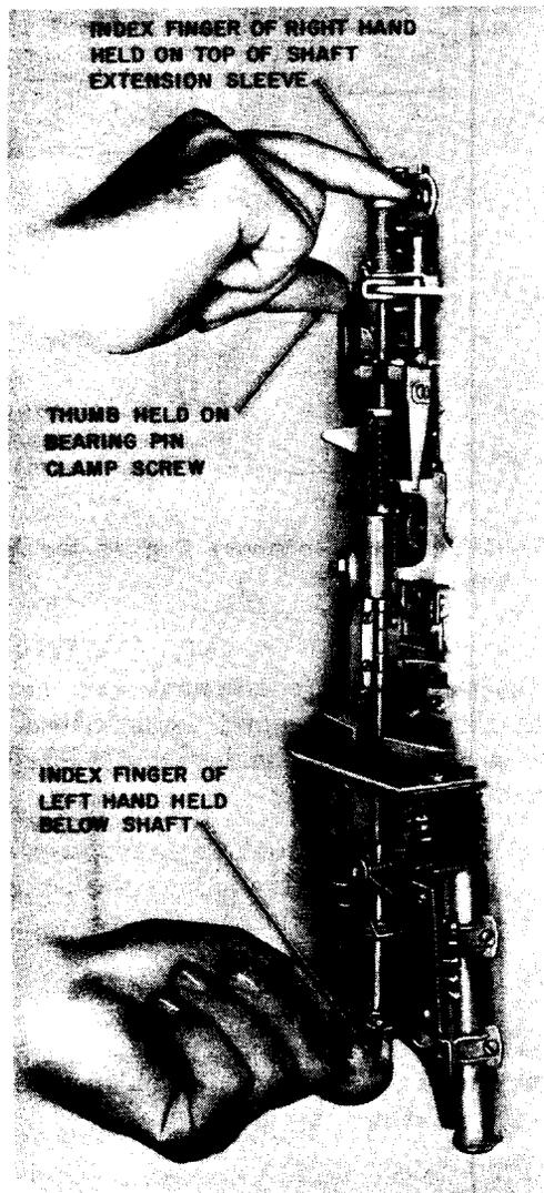
Fig. 25—Method of Raising Shaft
