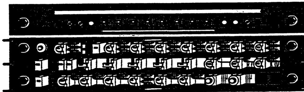
Figure 18. View of a Portion of a Power Board. Top is View of Ringling Generator Alarm Lamps and Control Keys. Bottom is View of Generator Hold-Up Relays (Cover Removed).
