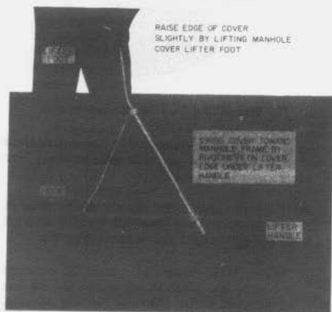
Fig. 42—Moving Cover to Manhole Frame
