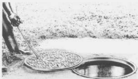
Fig. 15—Sliding G or H Cover Clear of Frame
