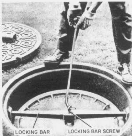
Fig. 27—Loosening Locking Bar Screw
