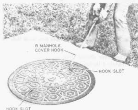
Fig. 12—Preparing to Unseat Type R Manhole Cover
