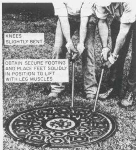
Fig. 34—Preparing to Unseat Cover—Two-Person Method
