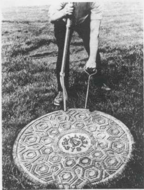
Fig. 31—Inserting B Manhole Cover Hook for Positioning on Locking Bar
