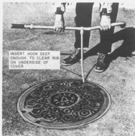
Fig. 29—Inserting PTS-49 Manhole Cover Lifter Hook Into Hook Hole
