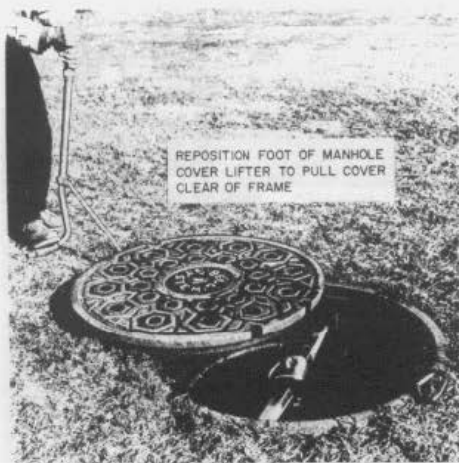
Fig. 33—Pulling Cover Clear of Frame
