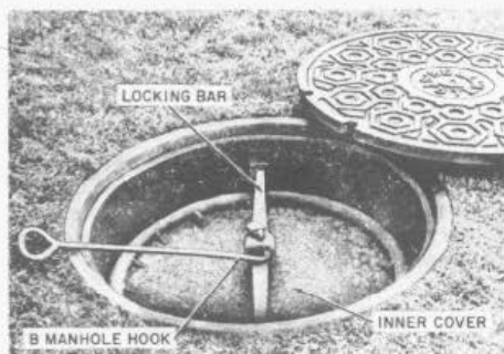
Fig. 2—Manhole Inner Cover
