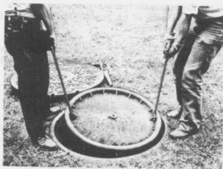
Fig. 38—Removing Inner Cover—Two-Person Method
