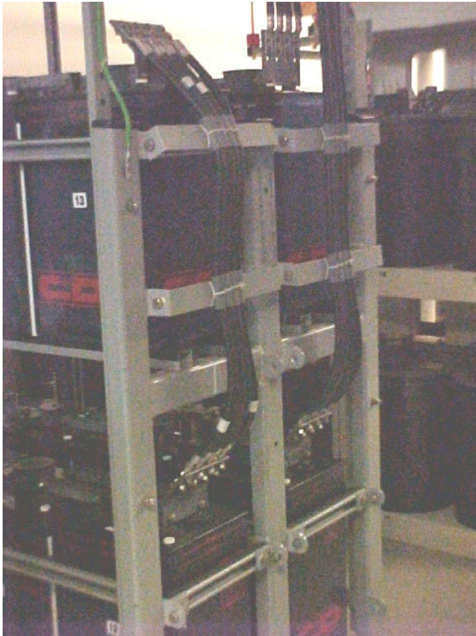
**Figure 2-4:** Typical Arrangement of Cables for A Battery Stand
