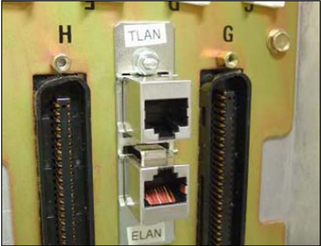
Figure 153 Installed Ethernet port adapter plate
