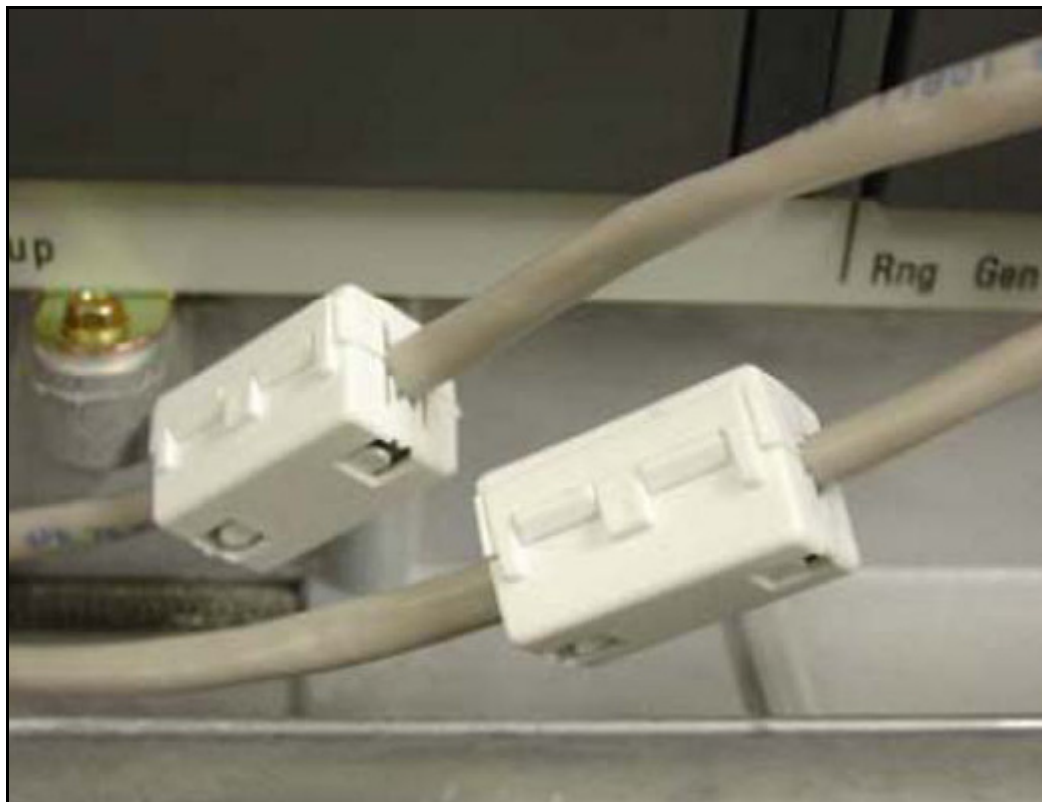
Figure 109 Attached Ethernet patch cable ferrite beads
