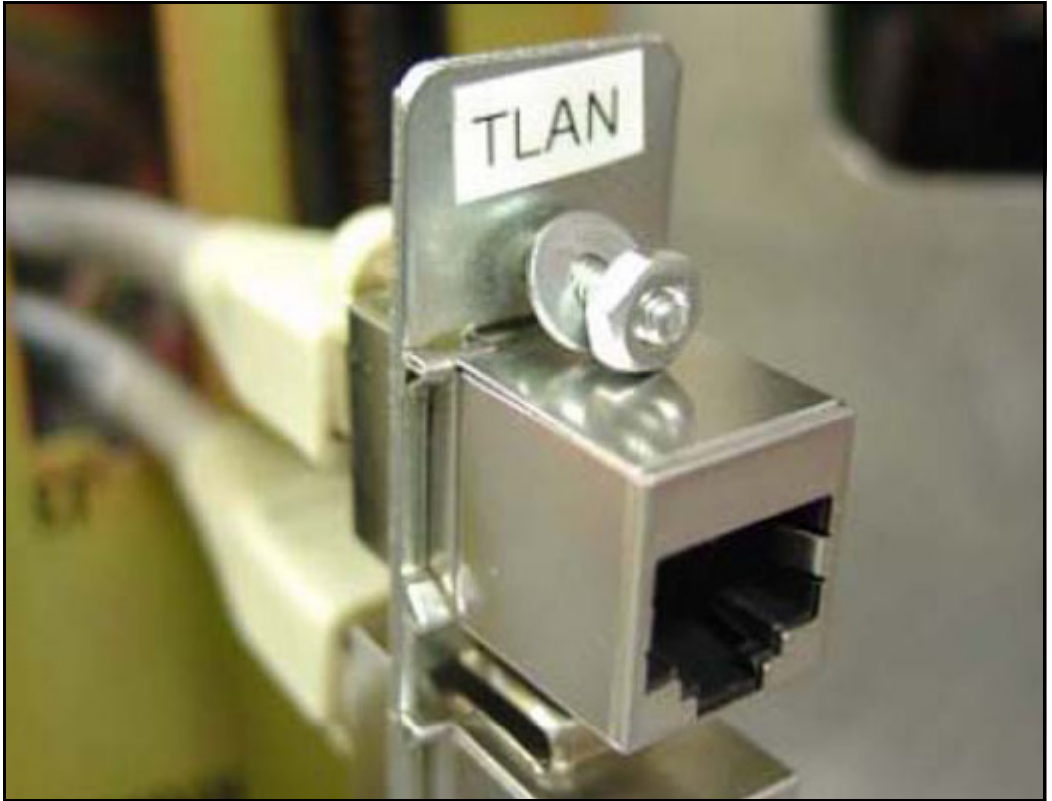
Figure 52 TLAN connection on Ethernet port coupler
