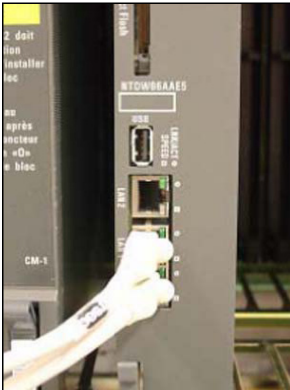
Figure 19 TLAN connection on faceplate
