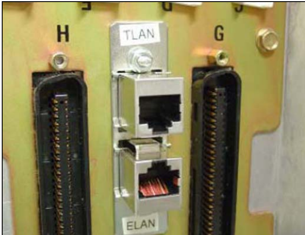
Figure 50 Installed Ethernet port adapter plate
