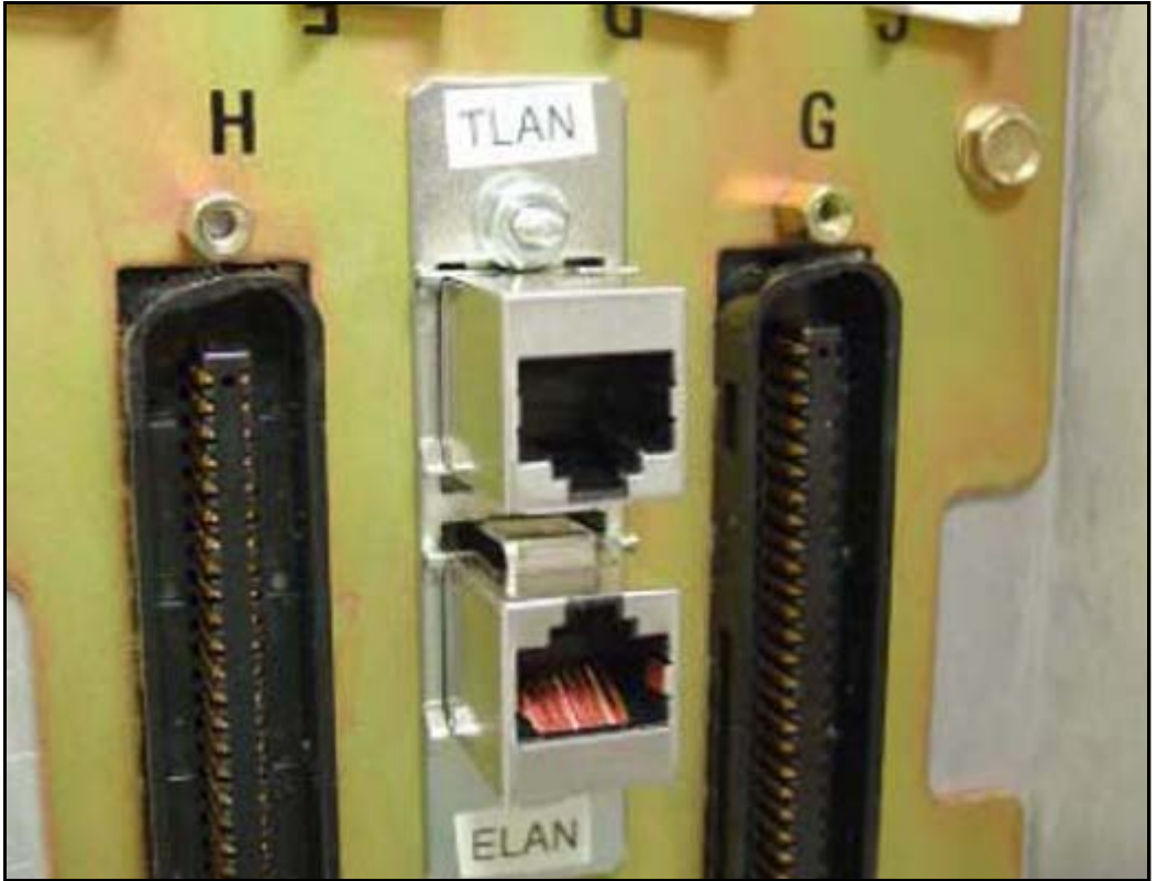
Figure 52 Installed Ethernet port adapter plate
