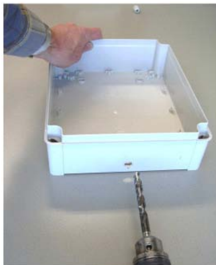
Figure 61: Drilling the hole (12 mm)
