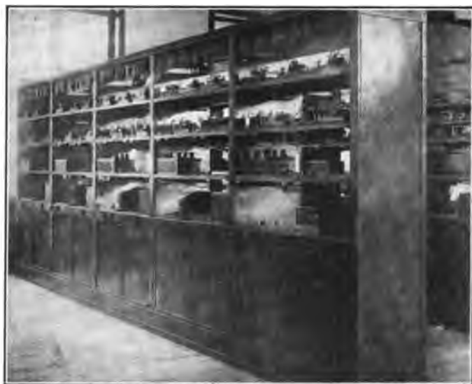
FIG. 357.—Multiplex repeater instrument rack used in "Postal" offices.
