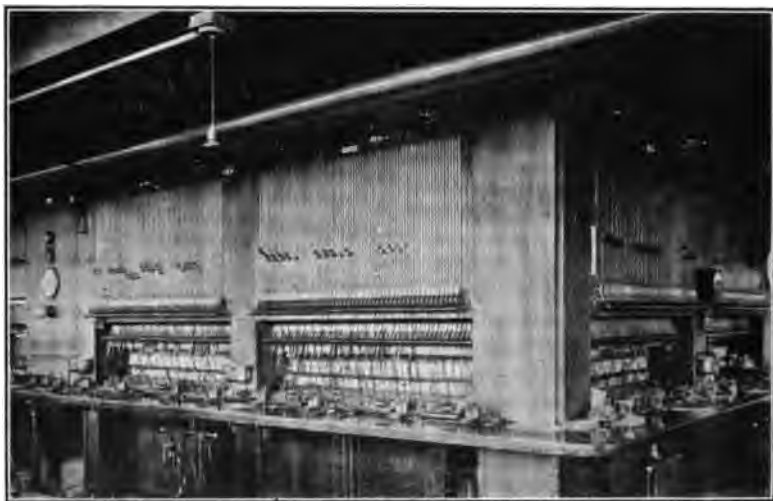
FIG. 131.—Sections of a main-line switchboard at a terminal office.
