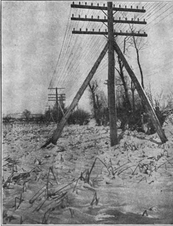
FIG. 142. — Effect of Sleet on a Properly Braced Pole Line.
