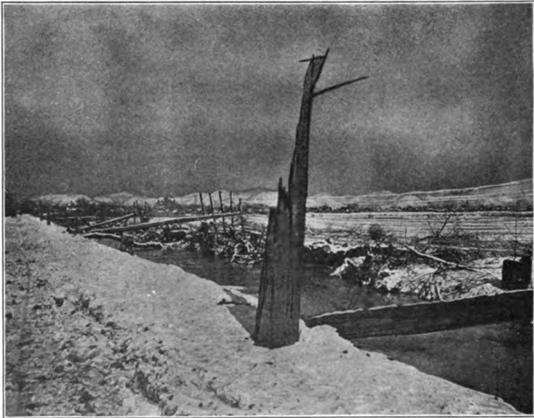
FIG. 139. — Effect of Sleet on Pole Line.
