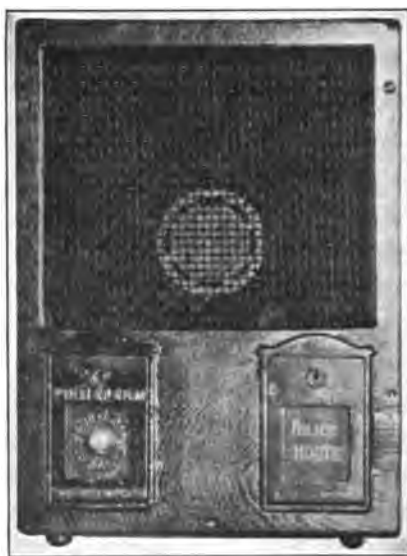
FIG. 165.—Fire and police box.
