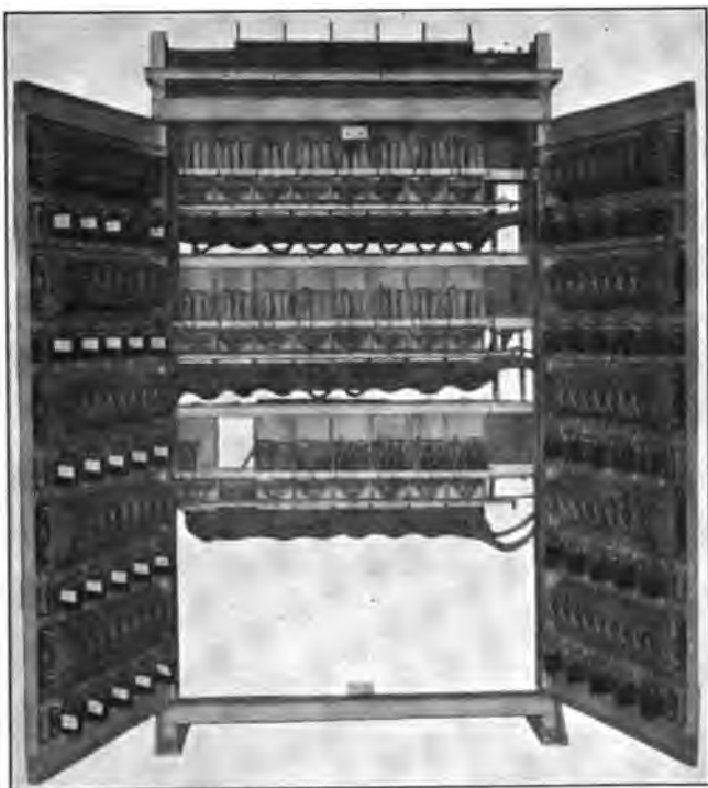
Fig. 89.—One-hundred-line switchboard, rotary lineswitches (front open).
