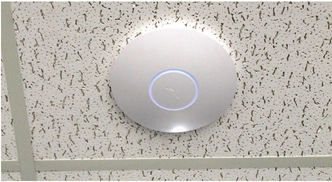
UniFi AP-PRO mounted on the ceiling
