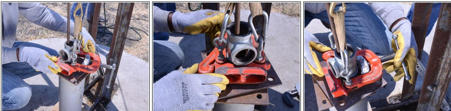
*(i)* This particular pump is using a tripod with a block and tackle to lift the riser main. C-wrenches may also be used to lift the riser main.
