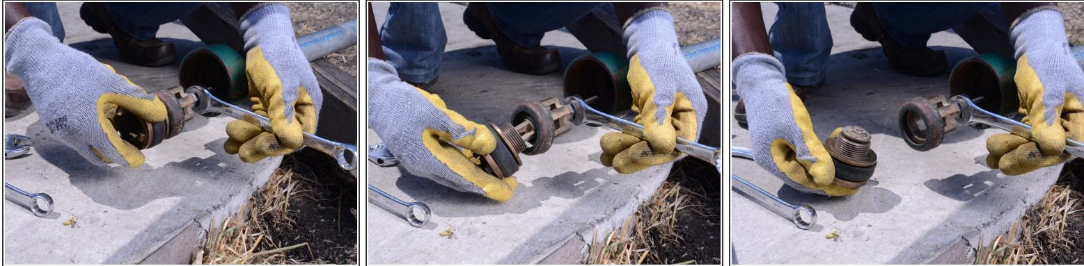
! Be careful to keep the valve parts off the ground.
