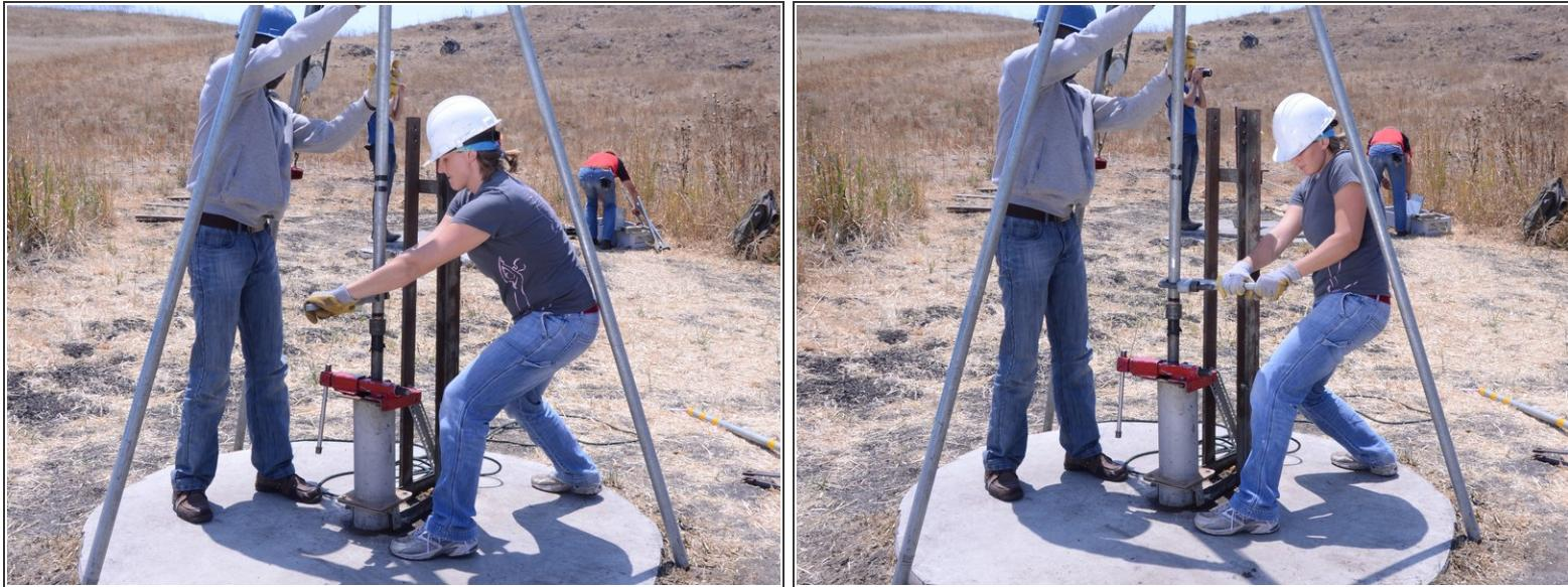
*(i)* Keep the pipe wrench a few inches above the joint in this step.
