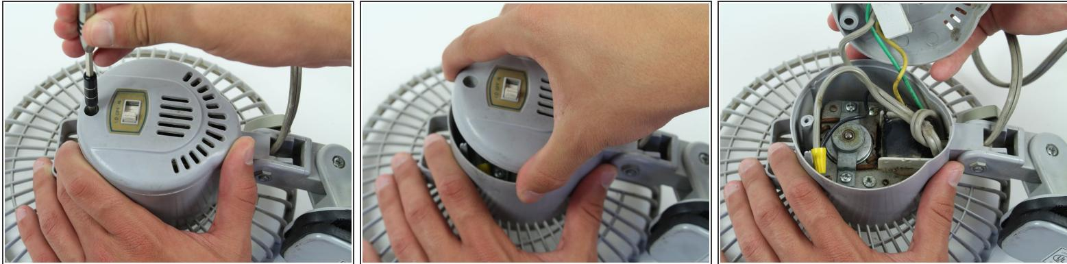
**⚠** Make sure to unplug the Comfort Zone CZ6C before replacing the motor. This will prevent the risk of electrocution.
