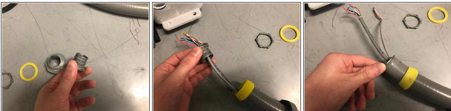
① Pull this piece over the wires and then screw it into the conduit
