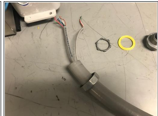
① Pull the cover over the conduit and the wires
