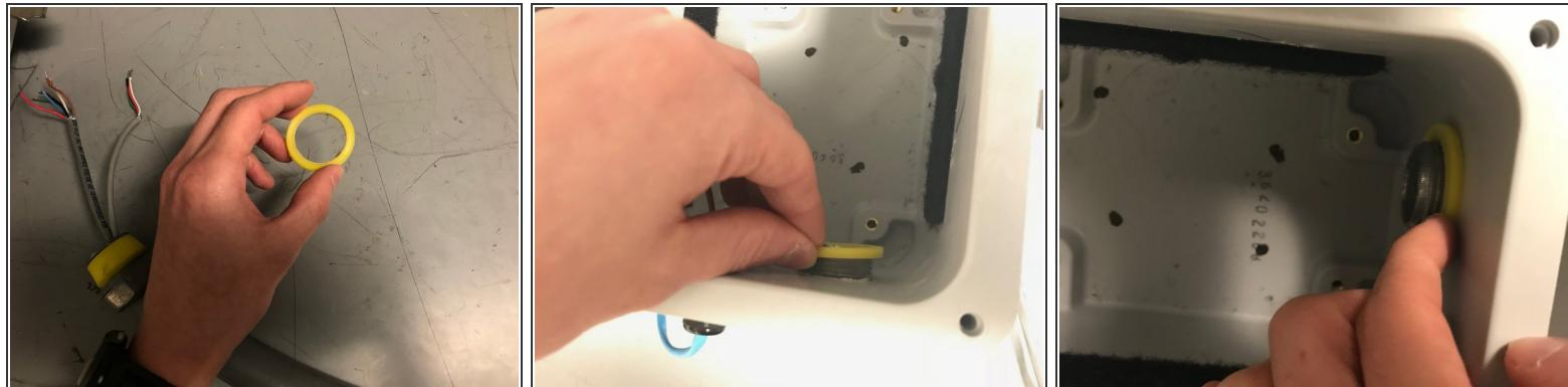
① Pull the yellow seal over the inside of the connector piece
