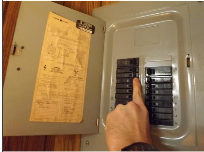
**⚠** Turn off electrical power from the breaker by switching off the breaker that is connected to the designated area.
