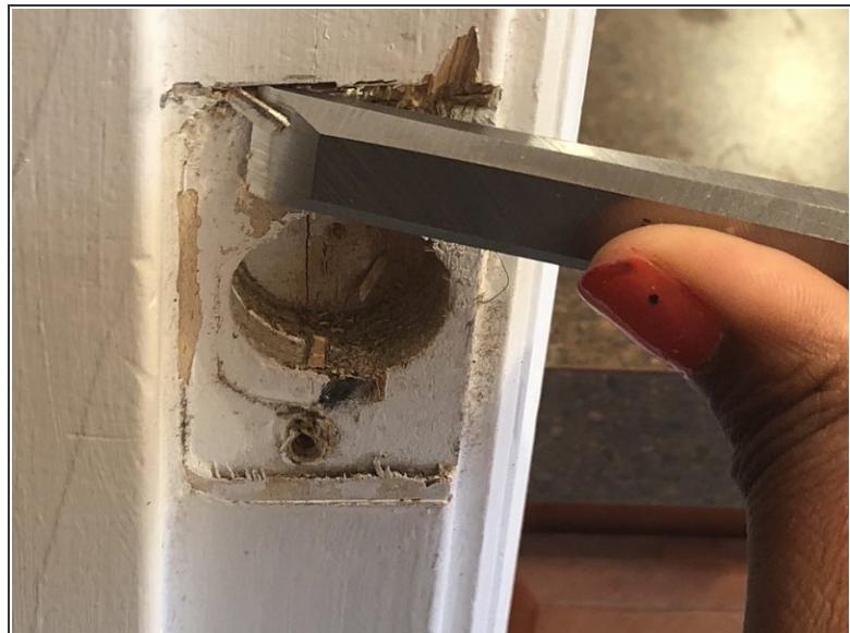
**⚠** Using the wood chisel, chisel out the wood above the line to make space for the new placement of the strike plate.
