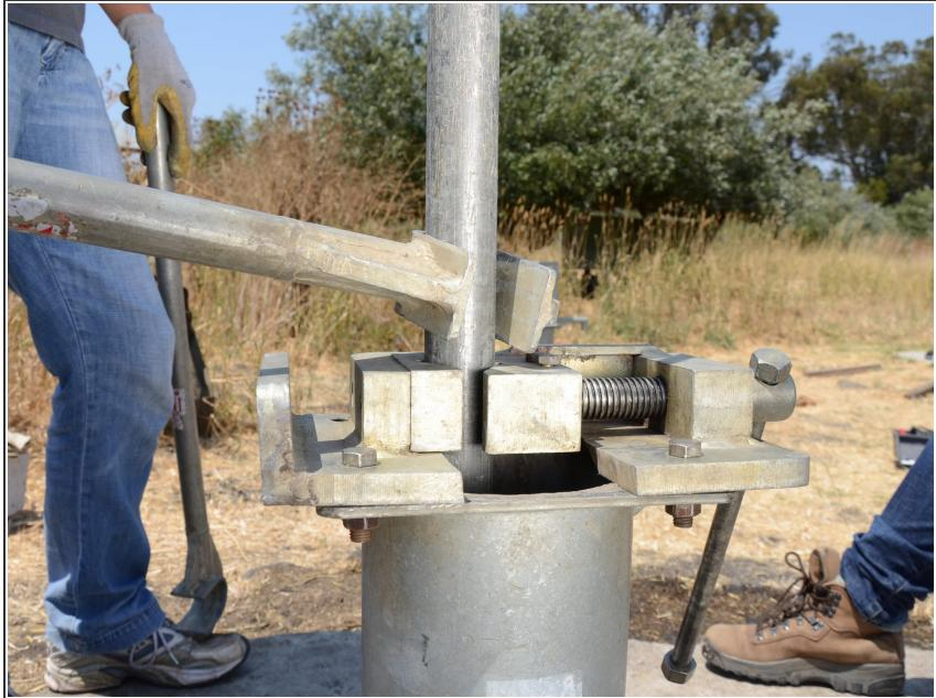
⚠ When using the lifting arms, it is essential that each arm have a gap above and below it, and that the openings alternate direction up the pipe.
