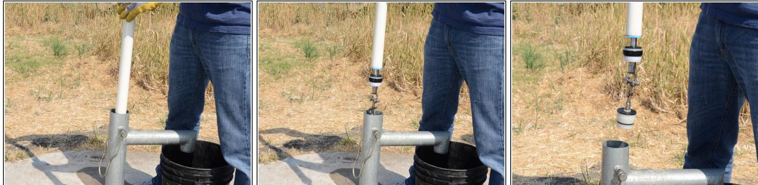
**i** The last section of riser main will have the traveling valve screwed on to the end, and the foot valve hooked onto the traveling valve.
