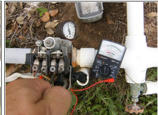
**⚠ WARNING:** The switch is supplied with 220V so one has to be careful not to get zapped. The first thing before doing anything is to flip the breaker to the pump switch and check it with a meter to ensure it is off.
